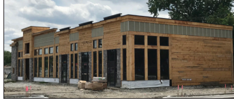
11650 S. Pulaski Firewater BBQ/Retail/Salerno’s Italian construction is underway.
